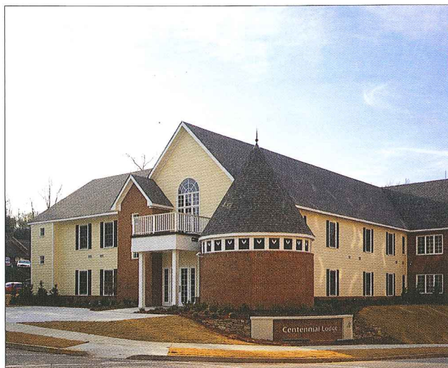
St. Vincent's Foundation built the Centennial Lodge as a gift to St. Vincent's Hospital during the hospital's 100th anniversary.
